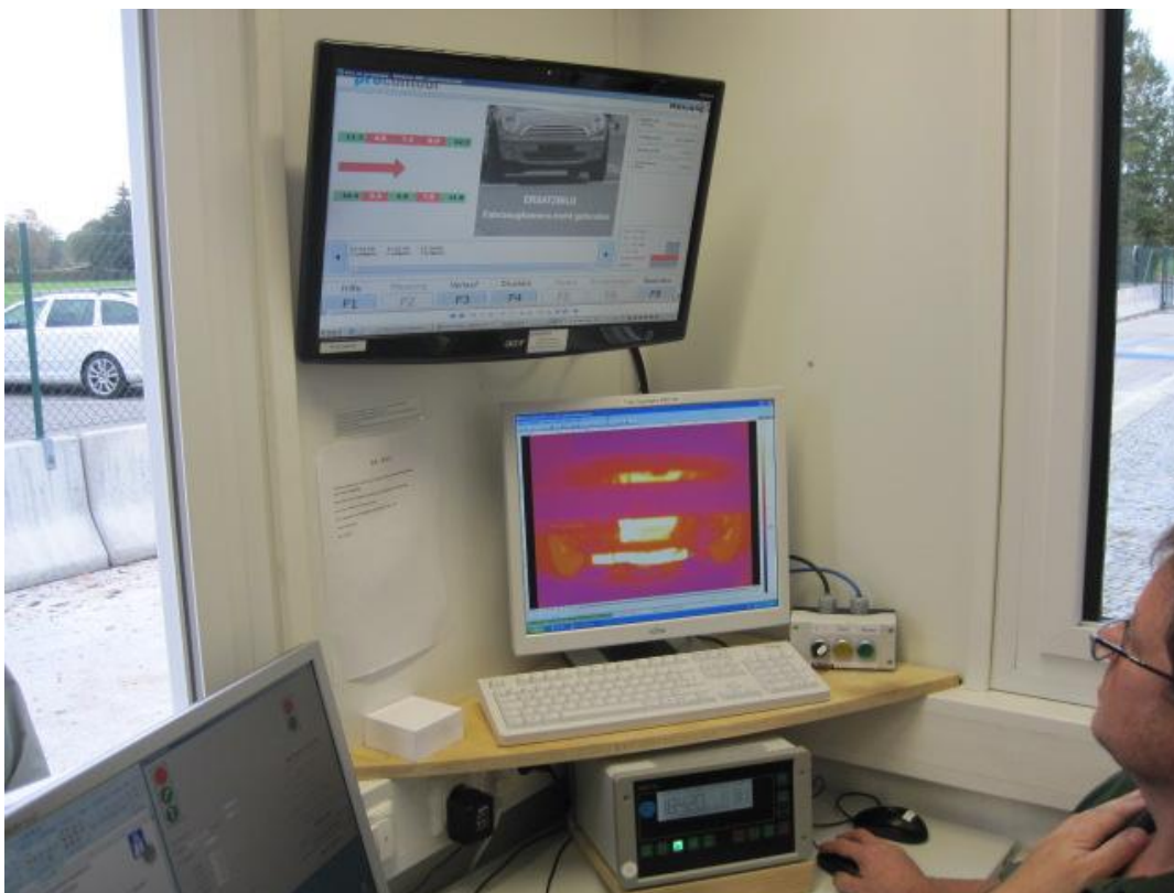
Figure 11 The thermal camera readout is on a separate screen in the control room.
