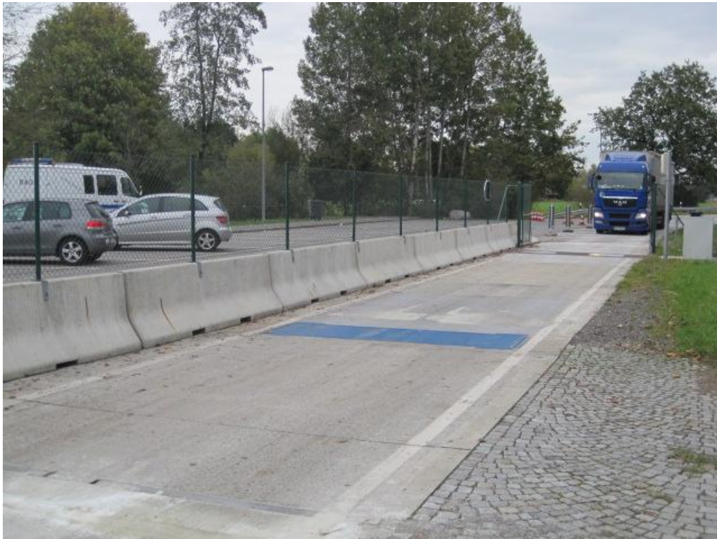
Figure 7 On the basis of screening or registration plate data, flagged vehicles are pulled out of traffic and into the lay-by by police, by traditional means
