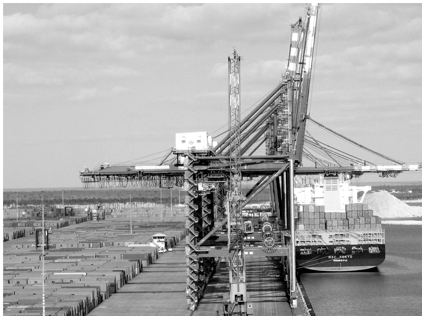
Figure 6 Gantry crane in a large container terminal (Photo: Linda Long)
