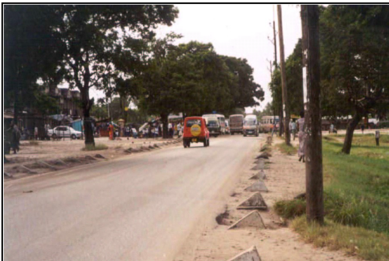
Figure 5. Triangular concrete bollards encourage vehicles to remain on the highway
