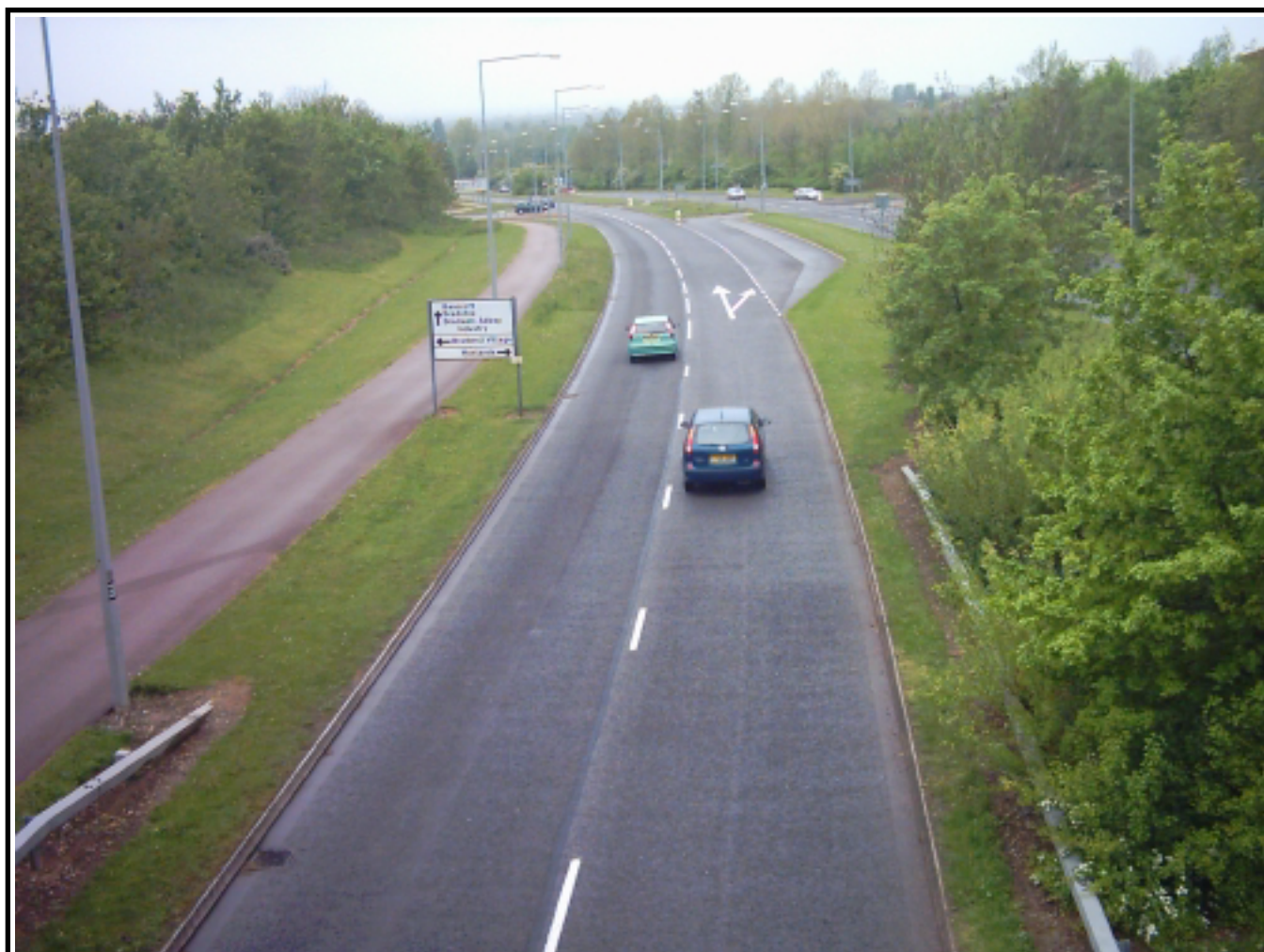
Figure 8. A highway designed for speed. Note that the bridge where the photographer is standing is protected from crashes by barriers. Note, too, how poorly the Redway is protected by a grass verge. Compare this with Tanzanian roads in Figure 6, 7 & 8 below [pp. 27, 28 & 29].
