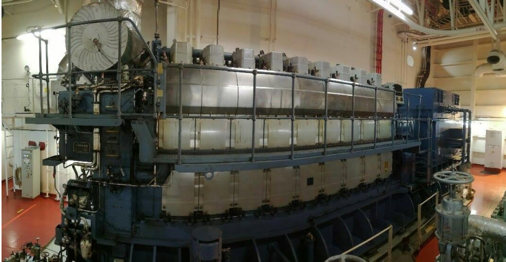
Figure 3. 11: Case ship's A/E with installed auxiliary EGE
